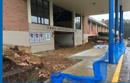
Demo of Main Entry Sidewalk & Brick Planter Walls
