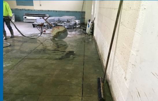
Sawcut Slab/Trenching to Install New Sewer Lines
