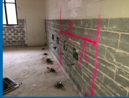
Exposing Existing Footing for New Elevator Pit/Shaft Footing
